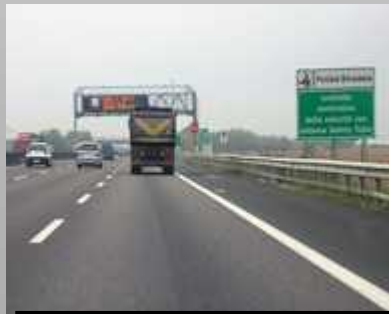
Highway data communications
