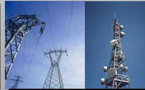
Energy transport data communications
